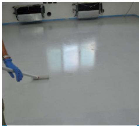
Finishing and waxing the surface
