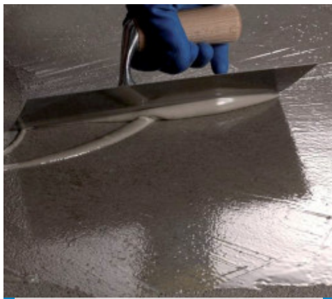
Priming the substrate
