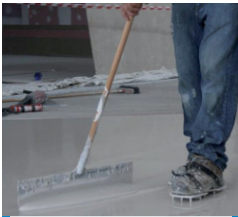
Application of self-levelling mortar
